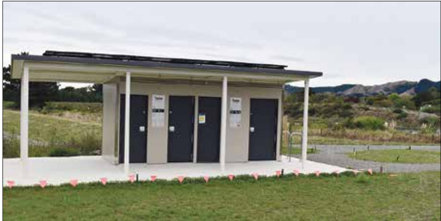
The toilets at Chrystalls Bend, closed until further notice. Photo Ōtaki Today
