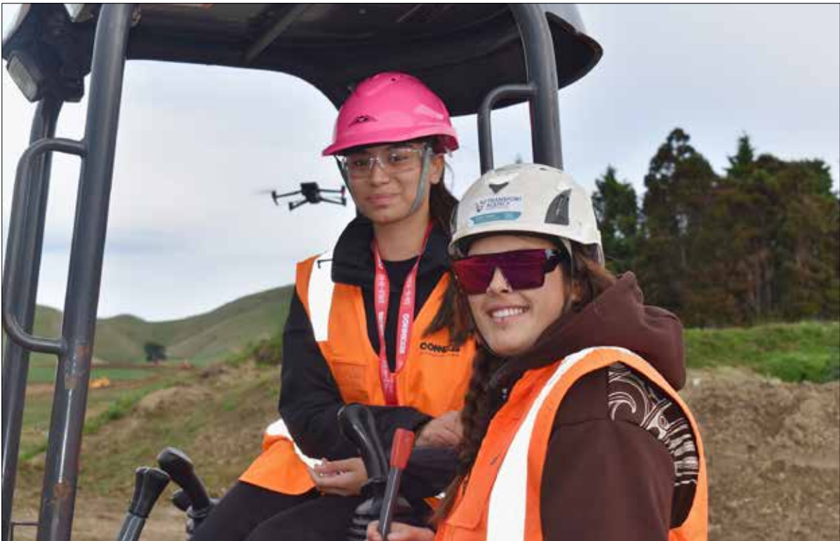
Okamanea Houia of Te Kura Kaupapa Māori o Te Rito tries her hand on a digger, watched by a drone and Downer Construction leading hand Hana Puketapu-Deyes. Photo Ōtaki Today
